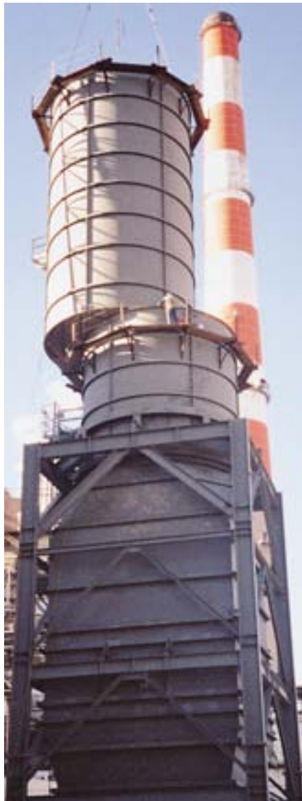
USA – SGT6-4000F exhaust system
