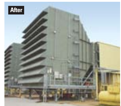
USA – 7B filter house retrofit
