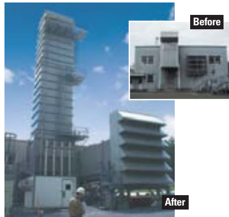
USA – FS5 filter house and exhaust system replacement
