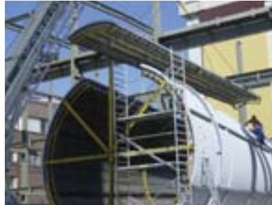
Italy – SGT5-4000F diffuser assembly
