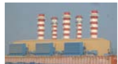
Qatar – 9FA exhaust system
