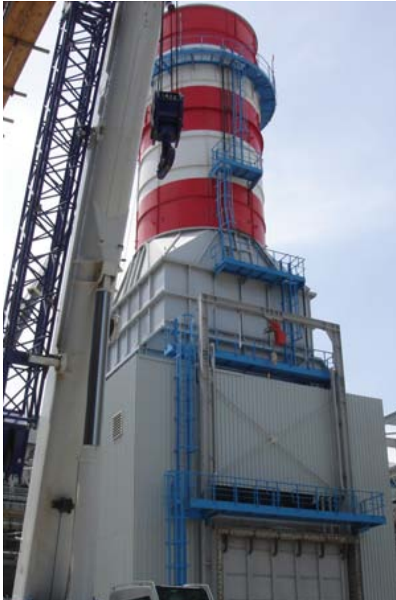
Qatar – SGT5-4000F diverter and exhaust system
