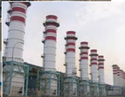
Indonesia – SGT5-3000E exhaust system
